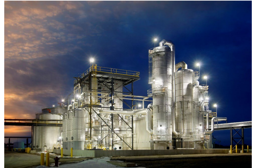
Figure 1: Evaporators and distillation columns at HCP
