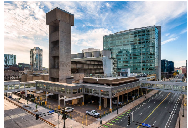
Minneapolis energy center (MEC)
