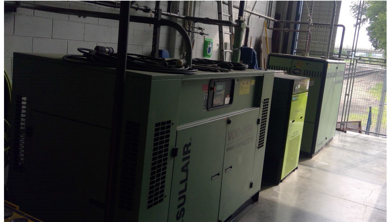
Air Compressors and Air Dryer
