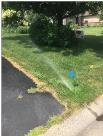
Before without a pressure-regulated spray head
