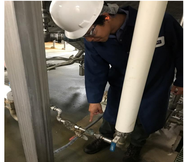
Orifice Steam Trap
