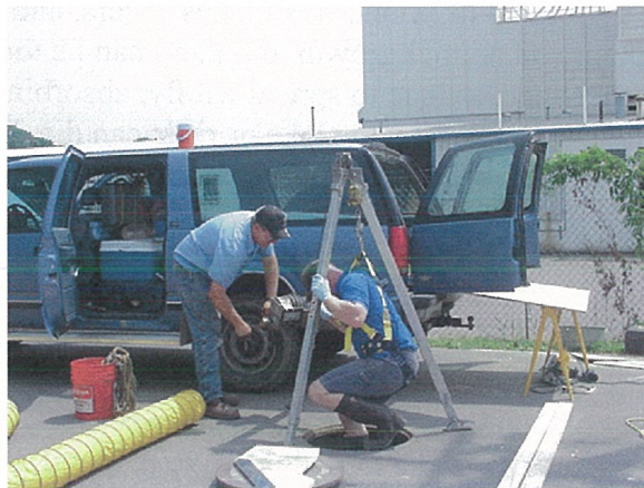
Figure 6: MVTL workers placing weir in manhole
